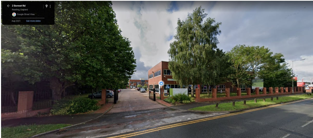
Above: Google Streetview image of the application site from August 2021, prior to the felling of trees within the application site along the Bennet Road frontage. Below: The existing context, subsequent to the removal of trees.
